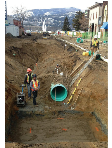
Excel makes sure that the Kelowna Lakeshore infrastructure project runs smooth and dry
