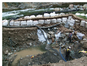
Excel does river diversions and dewatering for new fresh water intake structures
