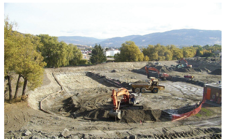
A perimeter dewatering system for the construction of a new waste water treatment plant in one of Excel's areas of expertise
